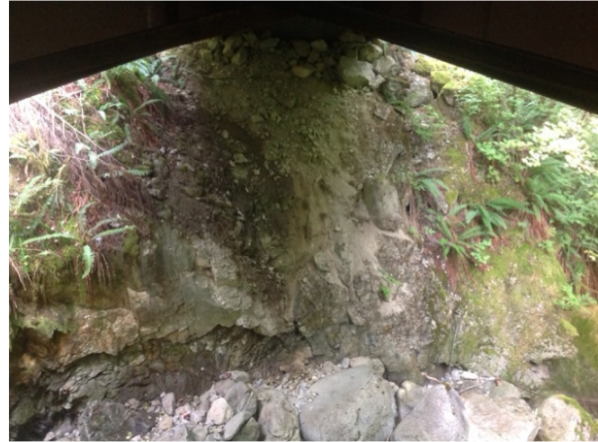
Left Bank Abutment when facing downstream
