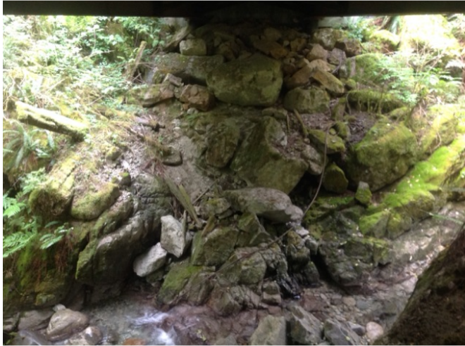
Right Bank Abutment when facing downstream
